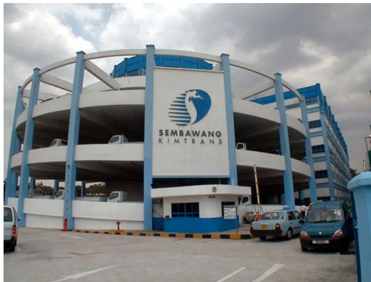
Figure 17.5: Multi-story warehouse with no automation but accessibility provided by a spiral truck ramp.
