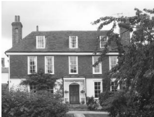
69 London Road, Tunbridge Wells
